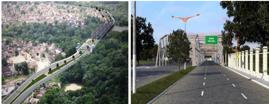
Figure 2. Areas that allows easy access of cars and people to APA Belém.
