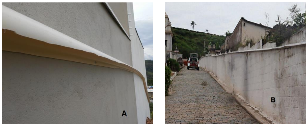
Figure 2 – Inverted PVC pipe structure installed around the municipal cemetery. (A) wall of property with installation of the device; (B) installation on the inside of the cemetery wall that borders houses. Municipal Cemetery of Serra Negra, state of São Paulo, 2024.
